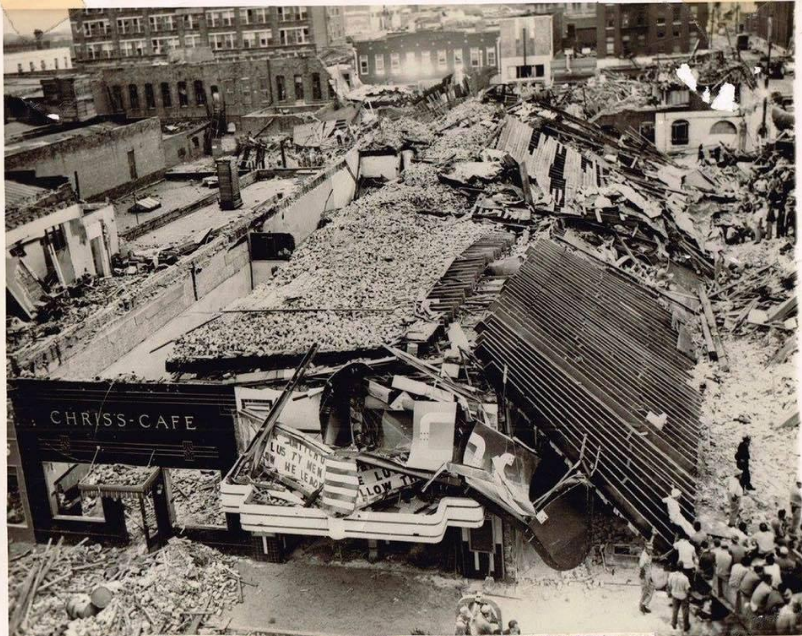
WACO, Texas, May 11, 1953--Bricks, beams and other debris
